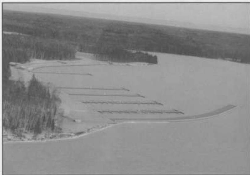
The construction of the new marina on Lake Waskesiu was the first time in the park's history that a major facility was not located at the townsite (credit: PANP)
