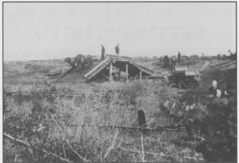
Loading gravel for the park highway (credit: NAC PA 164349)
