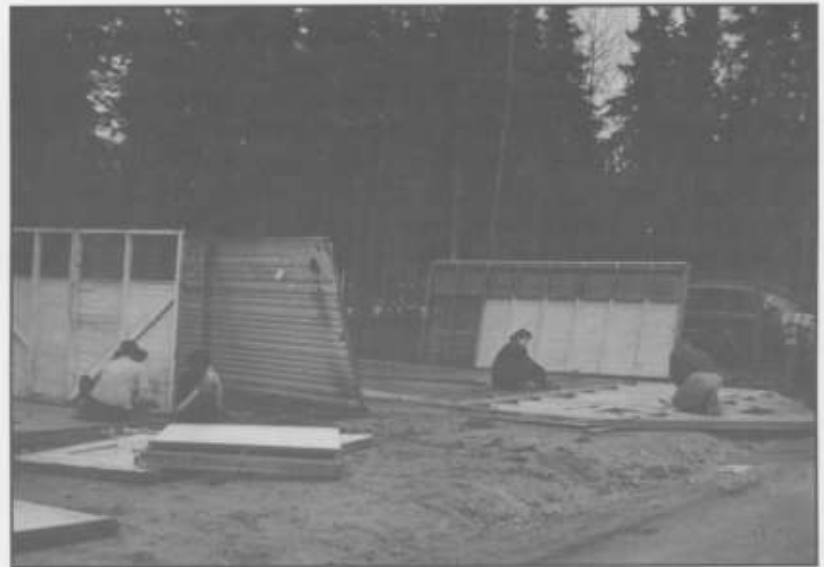
Erecting shack tents in the Waskesiu campground in the early 1960s (credit: Prince Albert Historical Museum)
