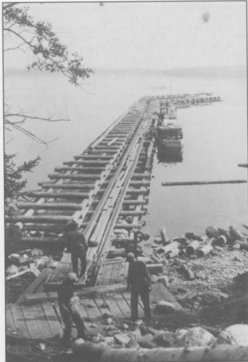
Alternate Service Workers placing rock in the new breakwater's cribbing, summer 1942 (credit: NAC C131588)
