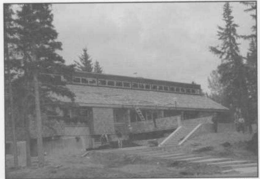
The new administration building enabled the park superintendent and office staff to work at Waskesiu year-round (credit: PANP)
