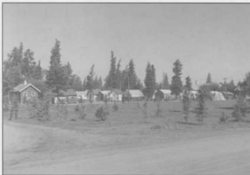
The Waskesiu shack tent community. (credit: SAB R-B2422(3))
