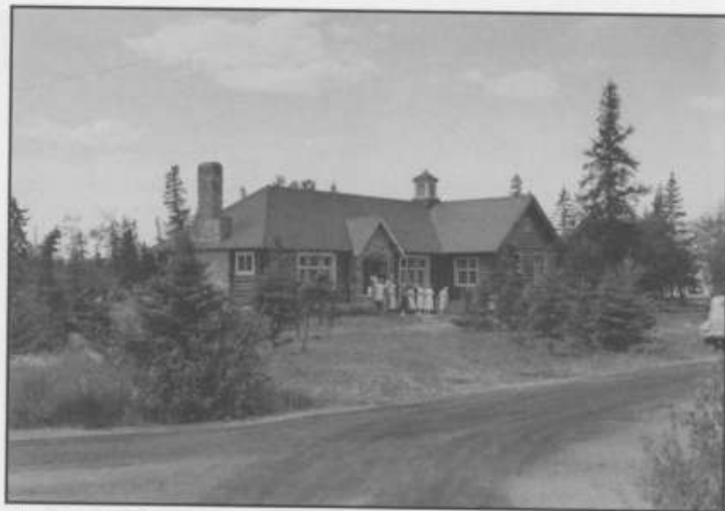
The Community Hall was enlarged in 1935 (credit: PANP 050-08)
