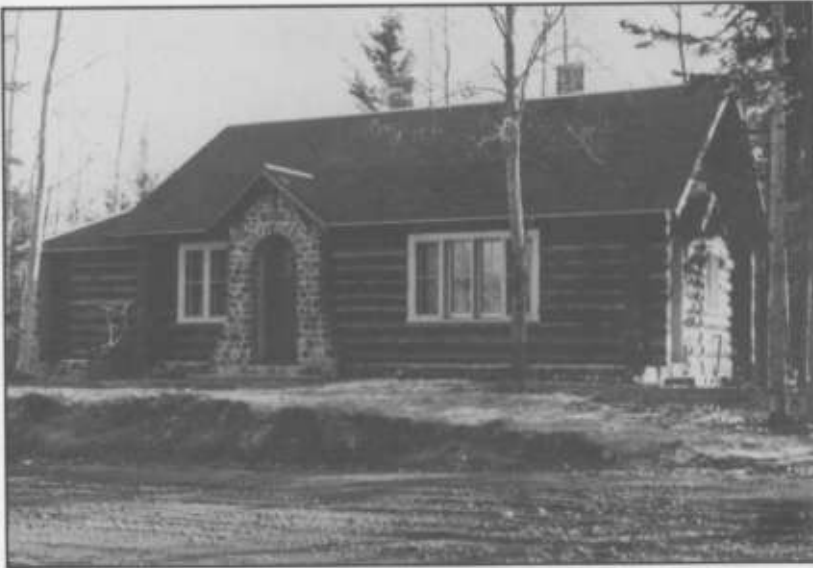
The RCMP building on the site now occupied by the Hawwood Inn (credit: NAC C131559)
