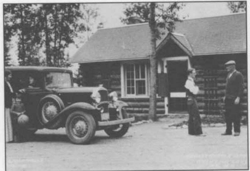
The Waskesiu campground registration office (credit: Friends of the Park [I. & E. Pease])
